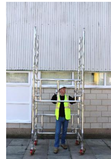
5. Fit 1 guardrail frame above the 7 th rung. Hooks facing outwards. (Refer to labelling to ensure that the frame is the correct way up)
