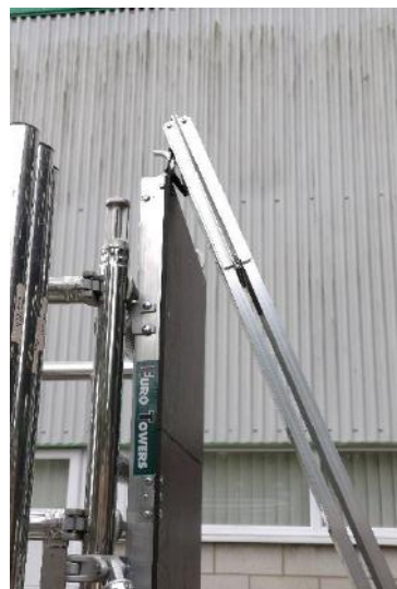
17. The toeboard can be located over the platform hook using the dedicated hanging strap.
