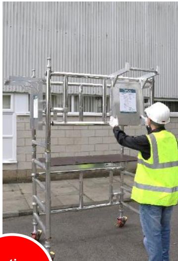
11. Remove toeboard and fit 2 assembly brackets in the position shown (side and front)
