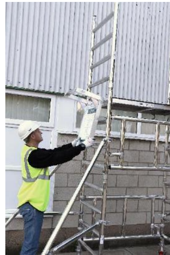
8. Fit an assembly bracket on the side of the tower.
