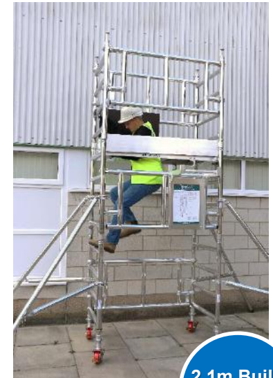
15. Access the platform using the trapdoor as shown and begin work.
