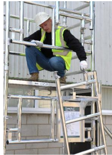
23. Retrieve 2 stowed side guardrail frames from the lower assembly bracket (front) pass them up to be relocated on the higher assembly bracket.
