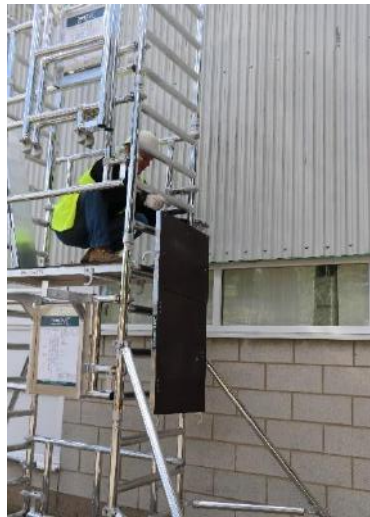
26. Remove the remaining platform from the lower section of the tower and pass up through the side frame.
