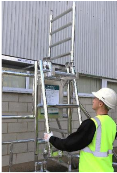
11. Stow the guardrail frames on the front assembly bracket.
