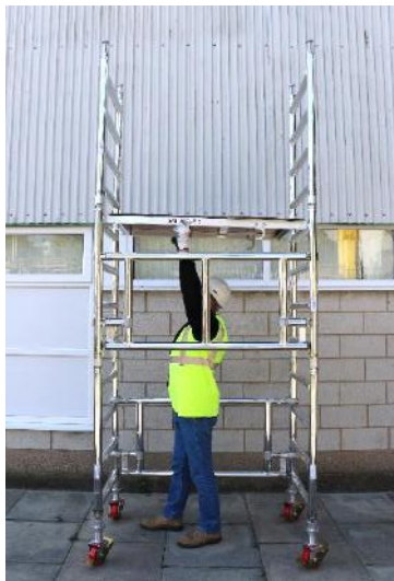
6. Fit the platform, 1 rung above the side frame location as shown.
