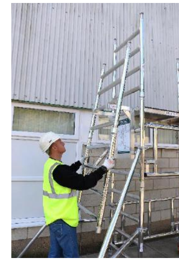
10. Stow the frames on the side assembly bracket
