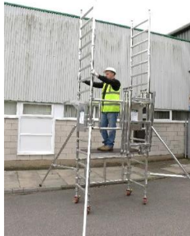
22. Repeat this process for the opposing side, ensuring that all interlock clips are engaged.
