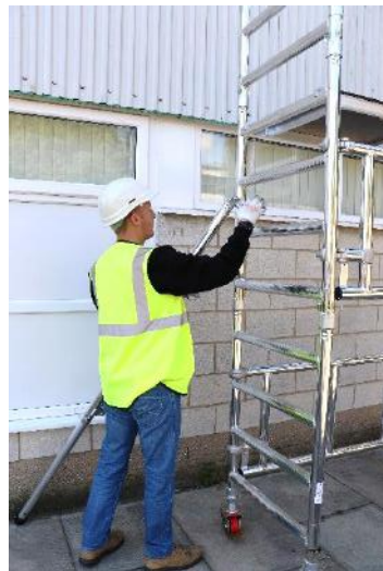
7. Fit 4 stabilizers, one on each upright of the tower.
