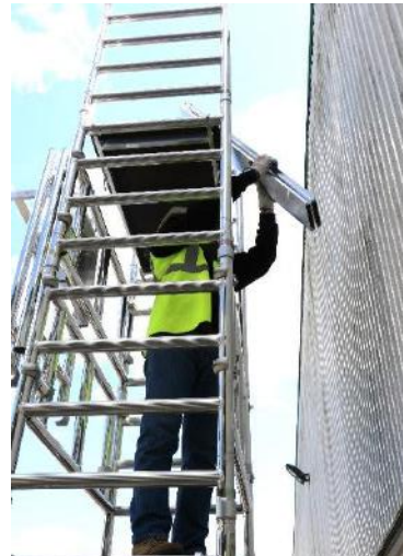
28. Relocate the toeboard assembly from the lower platform to the higher level, ensuring that it is positioned on the plain section of the platform as shown.
