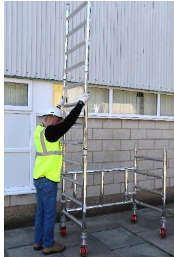
3. Connect 2 frames together and fit onto the base section at each end.
