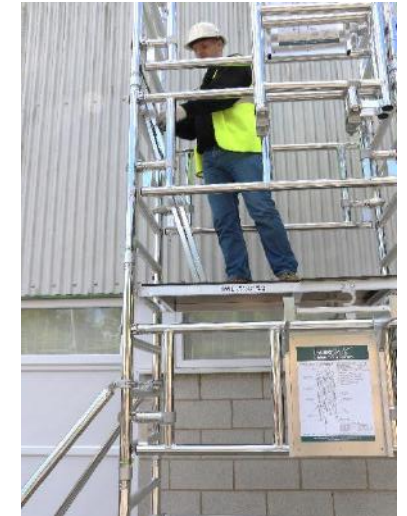
25. Temporarily locate the toeboard assembly on the platform to allow access to the additional platform that is stowed.
