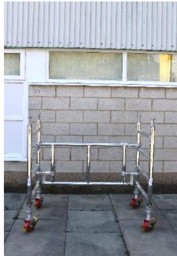
2. Fit a guardrail frame to the vertical member above the 3 rd rung with the hooks facing outwards.
