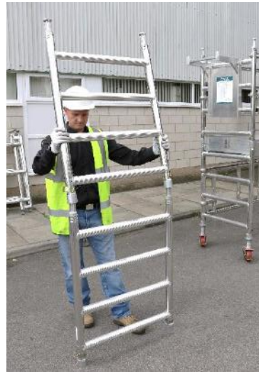
12. Assemble the frames in pairs as shown.
