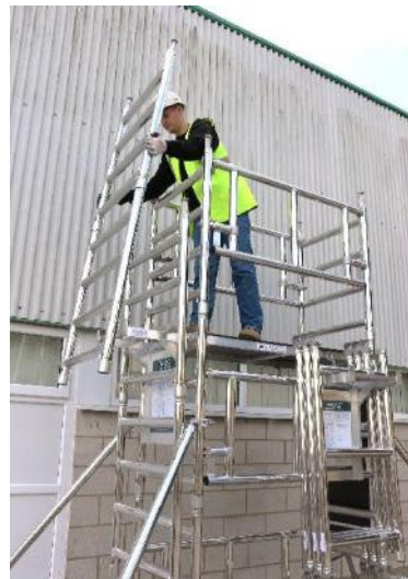
17. Retrieve a set of frames from the side assembly bracket and fit.
