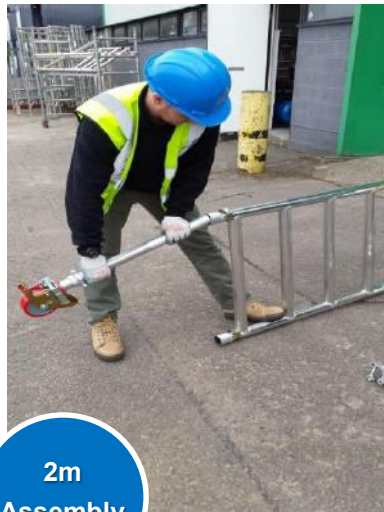
1. Insert legs and castors into a pair of frames.
