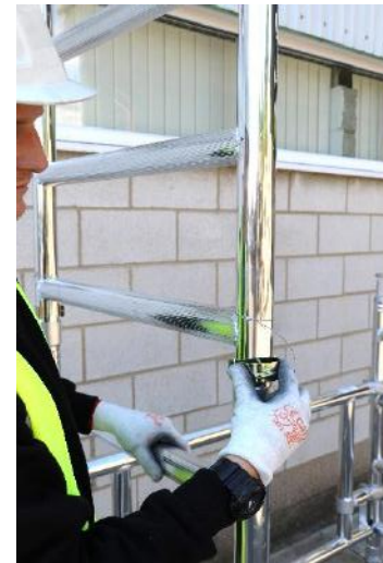
4. Engage interlock clips.
