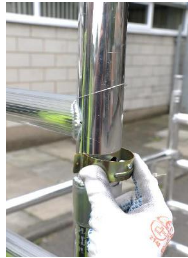
13. Engage interlock clips.
