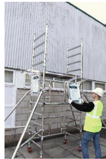
9. Fit the additional assembly bracket on the front of the tower as shown.
